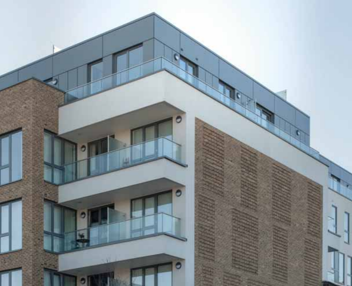
Project: Glenthorne Road Client: UK Facades Photo by Jim Stephenson Architect: Twenty First Architecture Ltd
