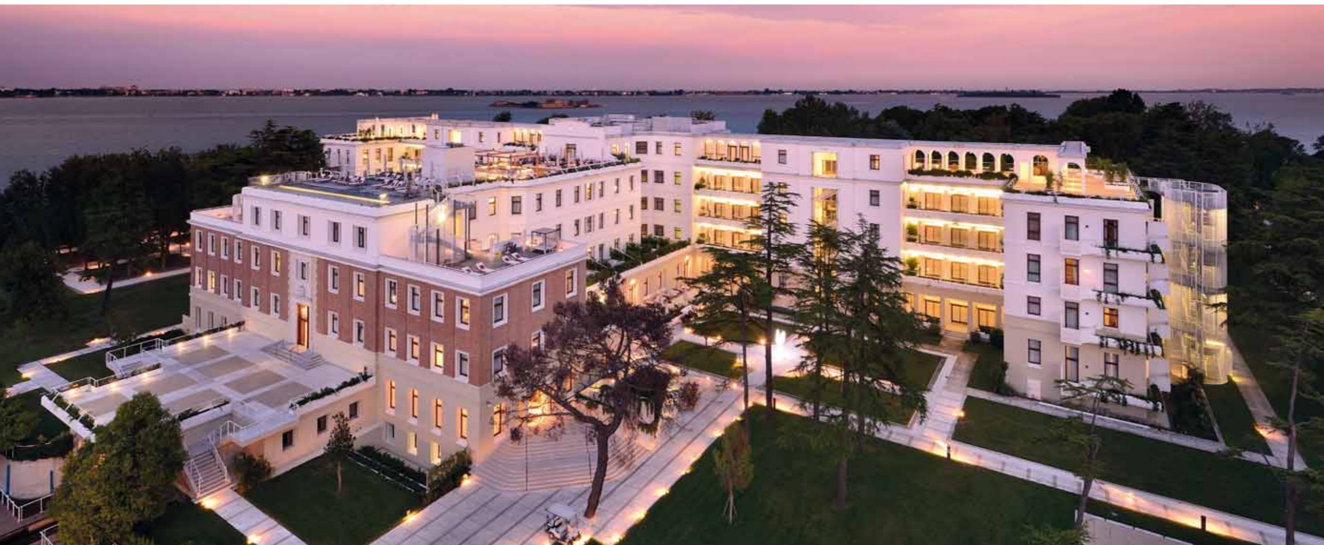
Project: JW Marriott Resort & Spa Isola delle Rose (Sacca Sessola) Venice Italy Client: Matteo Thun & Partners Architect: Luca Colombo MTL
